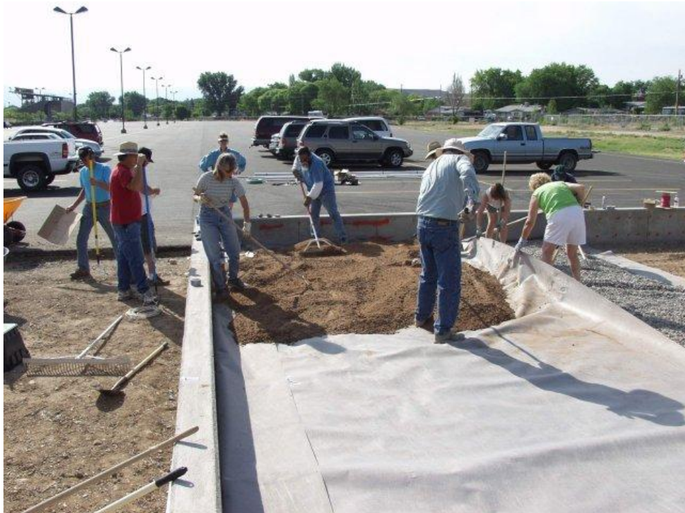
Applying washed round stones/gravel over the bottom layer of fabric
