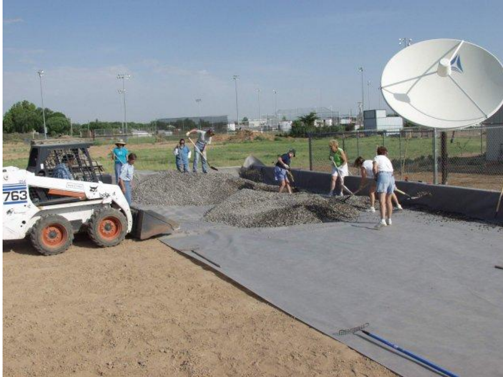
Applying washed round stones/gravel over the bottom layer of fabric
