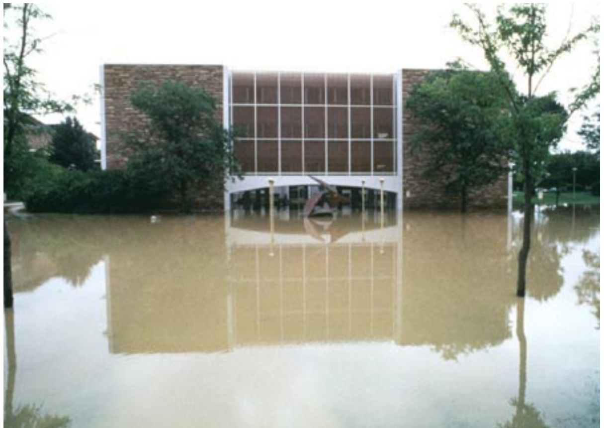
Inundated: The west side of Eddy Hall resembled a lake on July 29, the morning after floods hit campus. The basement of the building was filled to the ceiling with water, damaging or destroying books and decades of research work and other material collected by members of the Department of Philosophy and the Department of Foreign Languages and Literatures. (Photo by Instructional Services)
