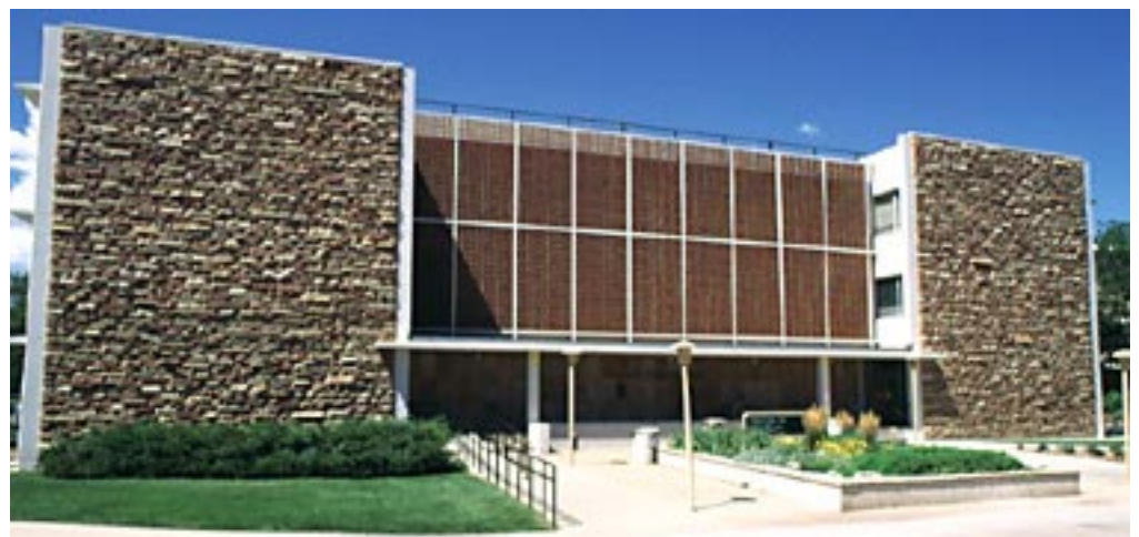
New era: In May, construction of classrooms, a writing center and computer instruction laboratories will be complete in the basement of Eddy Hall. (Photo by Bill Cotton)
